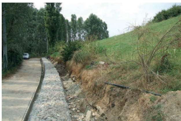
FIGURE 6: After the demolition of the wall, a permeable containment gabion is realized.
