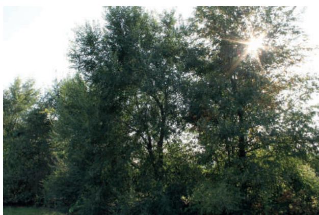
FIGURE 8: The absence of a waterproof sheet in the capping has allowed the growth of trees without compromising slope stability.
