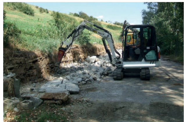
FIGURE 5: Demolition of the perimetric concrete wall.
