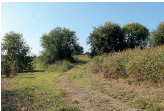
FIGURE 4: The layer of soil reported on the capping proved to be suitable for the growth of even tall trees.
