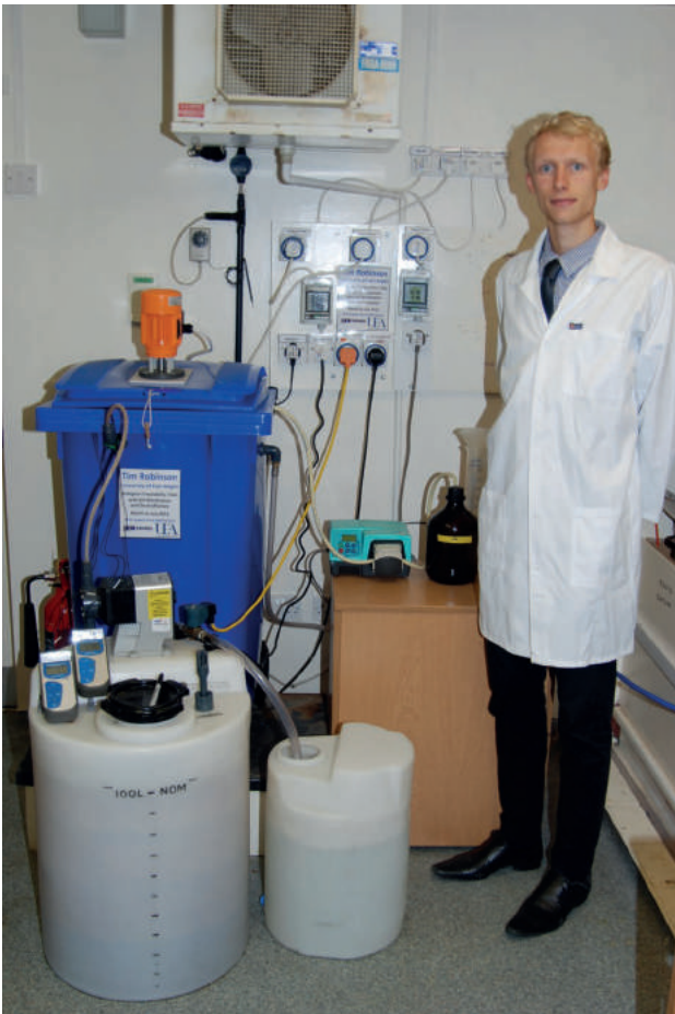
PLATE 2: View of the experimental units, showing feed tank and dosing pump, the 240 litre SBR reactor, electrical control panel, and treated leachate tank.
