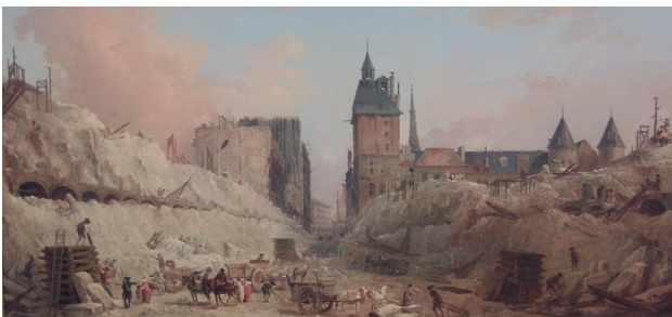
HUBERT ROBERT / Demolition of houses on The Pont au Change (1788).
