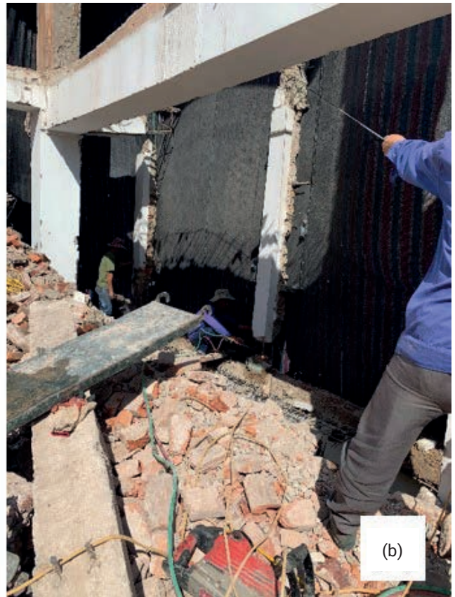
FIGURE 8: (a) Demolition by handheld tool; and (b) A worker manually pulling down an RC column.
