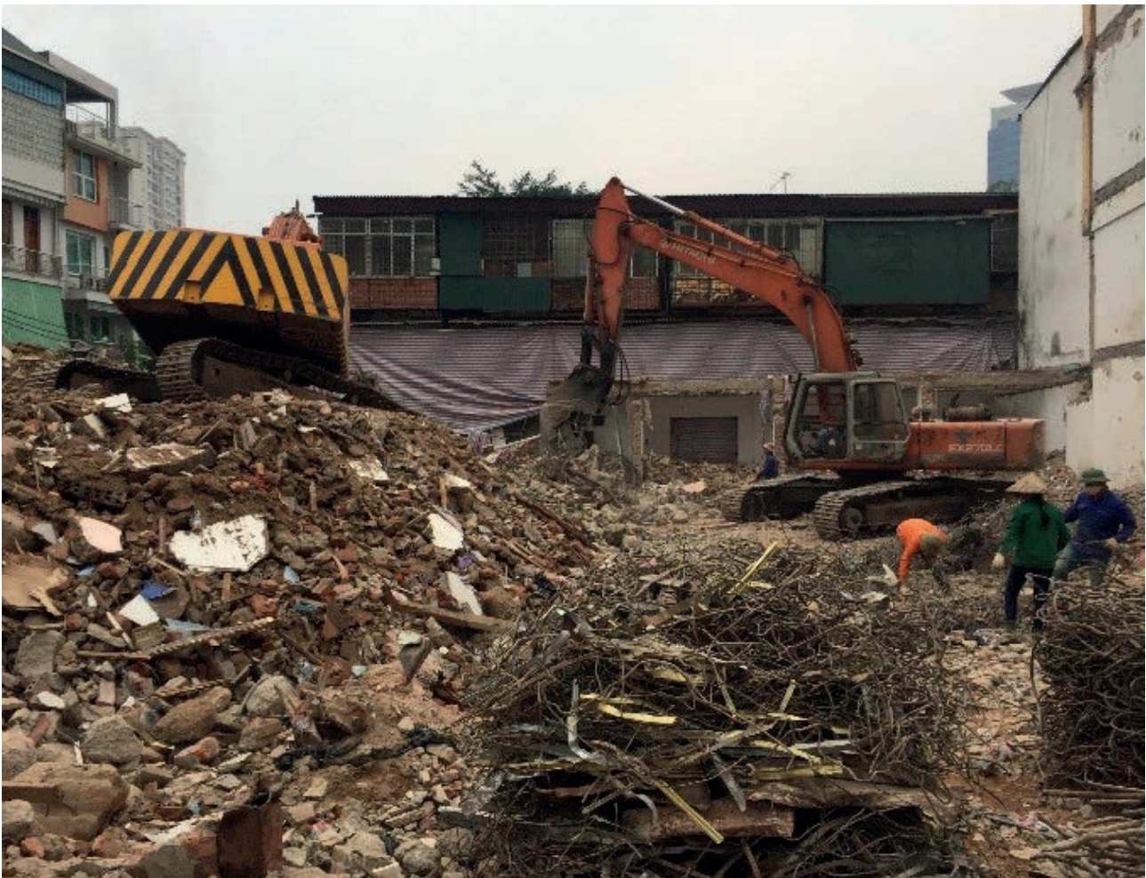
FIGURE 11: Reinforcing steel being separated and recollected.
