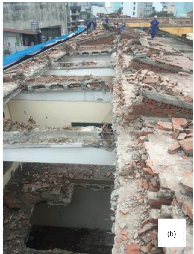
FIGURE 9: (a) Hole for CDW to fall through; and (b) Edge slab panels demolished.
