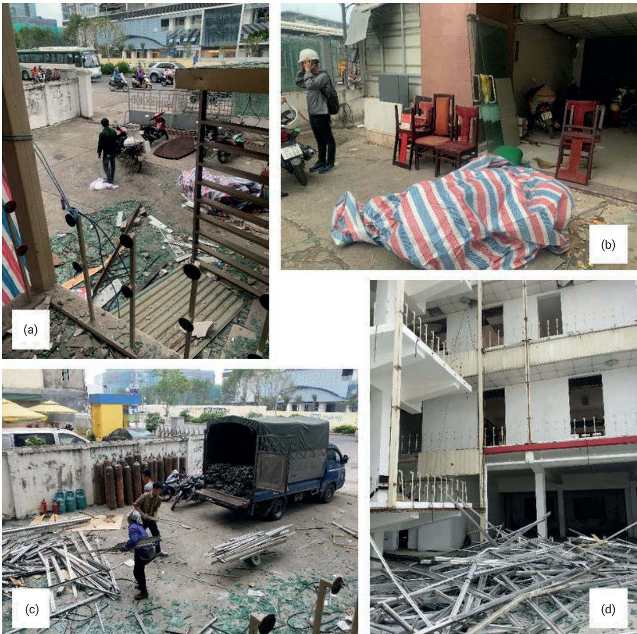
FIGURE 7: Removal of (a) sanitary ware; (b) interior furniture; (c) and (d) aluminum façade at OFC-01.
