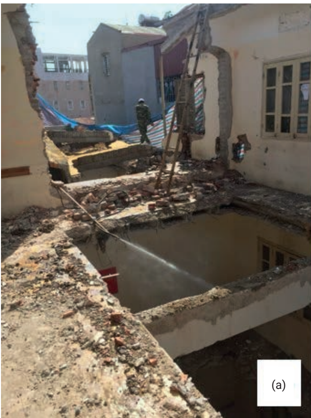
FIGURE 9: (a) Hole for CDW to fall through; and (b) Edge slab panels demolished.
