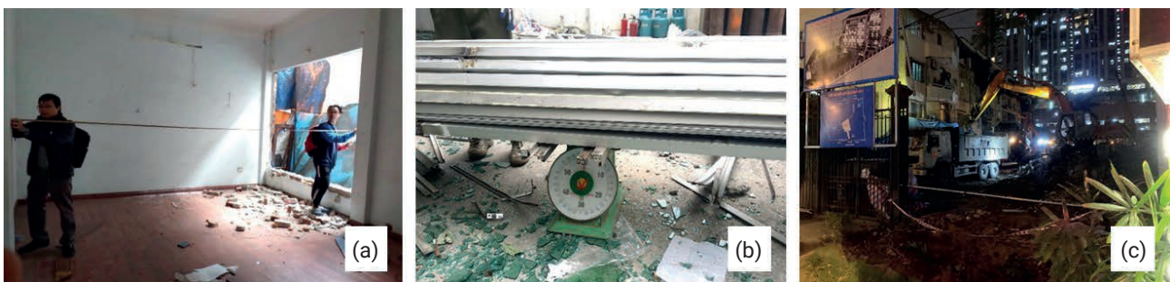
FIGURE 1: Survey of CDW generation (a) Determining GFA; (b) Scrap buyers measuring the amount of aluminum; and (c) Counting the number of CC-CB transport trucks.
