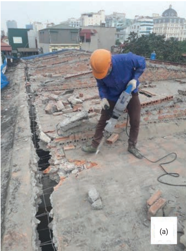
FIGURE 8: (a) Demolition by handheld tool; and (b) A worker manually pulling down an RC column.
