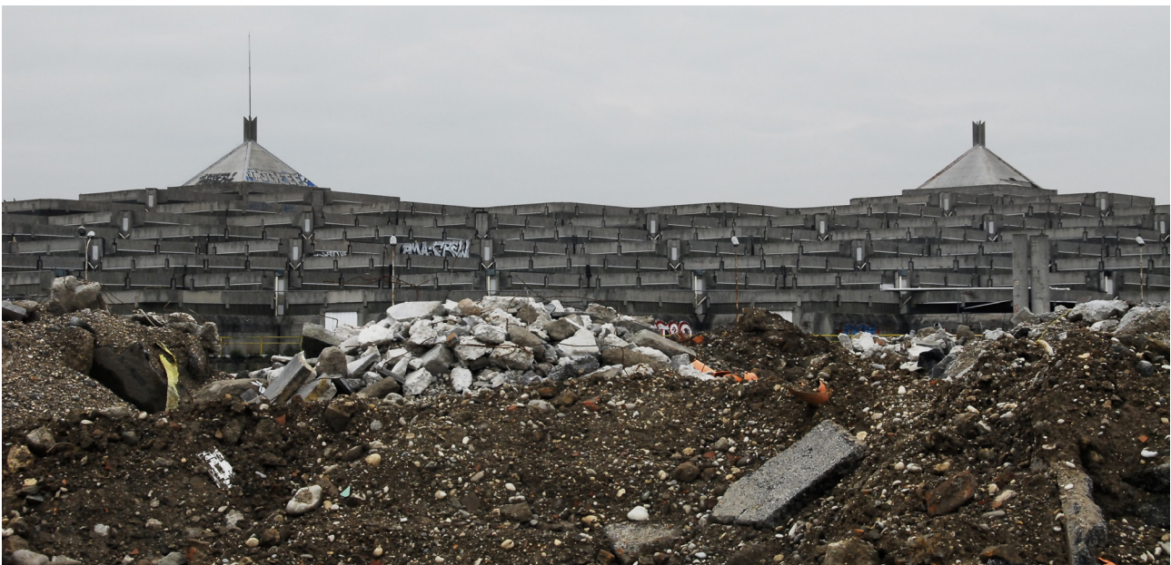
FIGURE 3: The Former Cattle Market of Padova (1967), by architect Giuseppe Davanzo (1921-2007). Photo by Stefanos Antoniadis, 2012.
