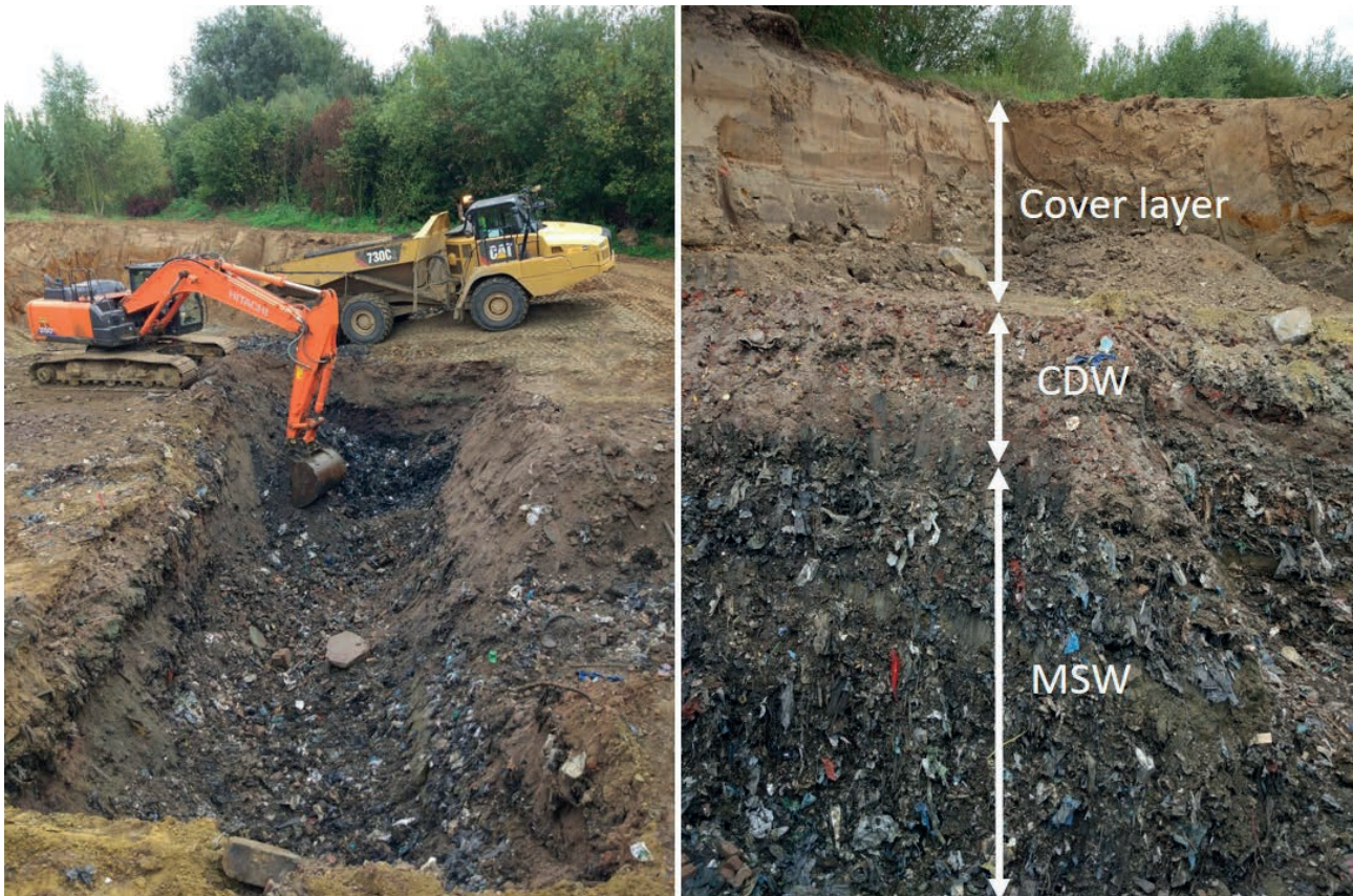
FIGURE 2: Excavation at the Mont Saint Guibert Landfill, Belgium.
