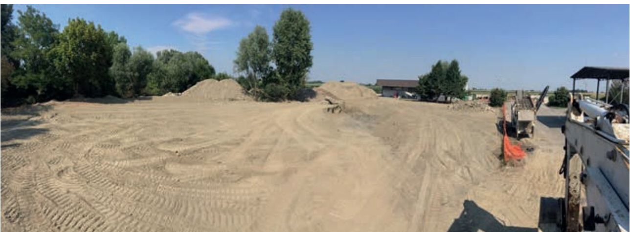
FIGURE 6: The landfill area before LFM intervention.
