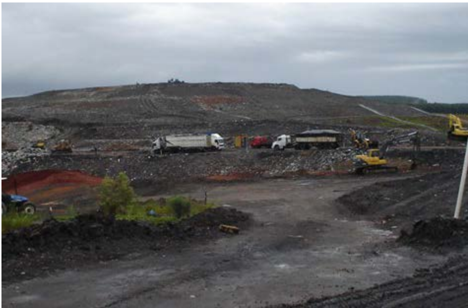
FIGURE 2: A daily service front of the landfill.
