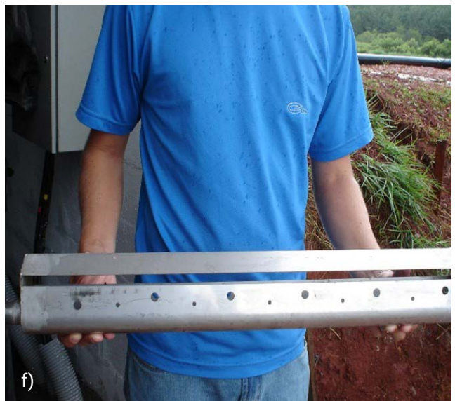
FIGURE 4: (a) Leachate distribution piping and concrete beams (to support the air piping); (b) spreading of gravel over the liquid distribution piping; (c) image of the blower house; (d) view of the air distribution piping installation assembly; (e) installation of the last sections of the air piping; (f) detail of the bubble diffuser.
