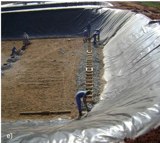
FIGURE 3: (a) Excavation and preparation of the base to begin construction of the filter; (b) start of installation of the waterproofing membrane; (c) welding of the membrane; (d) image of the progress of the waterproofing work; (e) preparation of forms for concreting the leachate pipe support; (f) spreading of gravel at the base of the filter.
