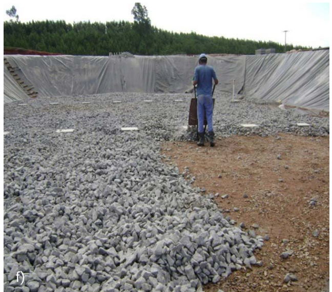
FIGURE 3: (a) Excavation and preparation of the base to begin construction of the filter; (b) start of installation of the waterproofing membrane; (c) welding of the membrane; (d) image of the progress of the waterproofing work; (e) preparation of forms for concreting the leachate pipe support; (f) spreading of gravel at the base of the filter.
