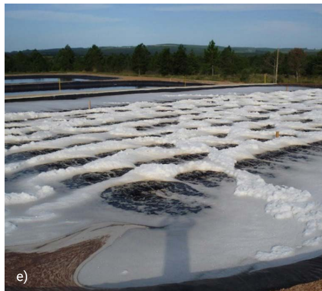
FIGURE 5: (a) Air distribution test and blower test; (b) filling the filter bed with gravel, after the successful aeration test; (c) another view of the air distribution piping, now with the filter completely filled with gravel; (d) view of the first author of this article, above the filter bed of the filter; (e) immediately after the beginning of operation at the filter.
