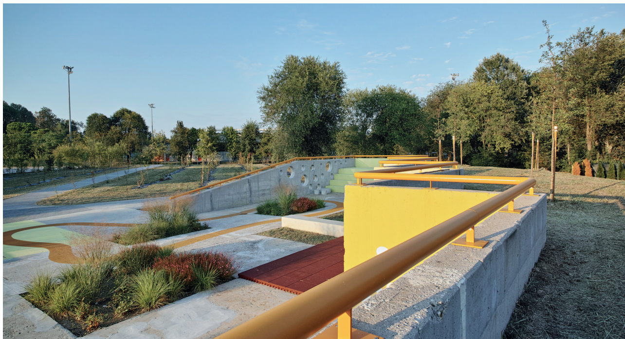
FIGURE 12: View from the top of the embankment towards the regenerated woodlands.
