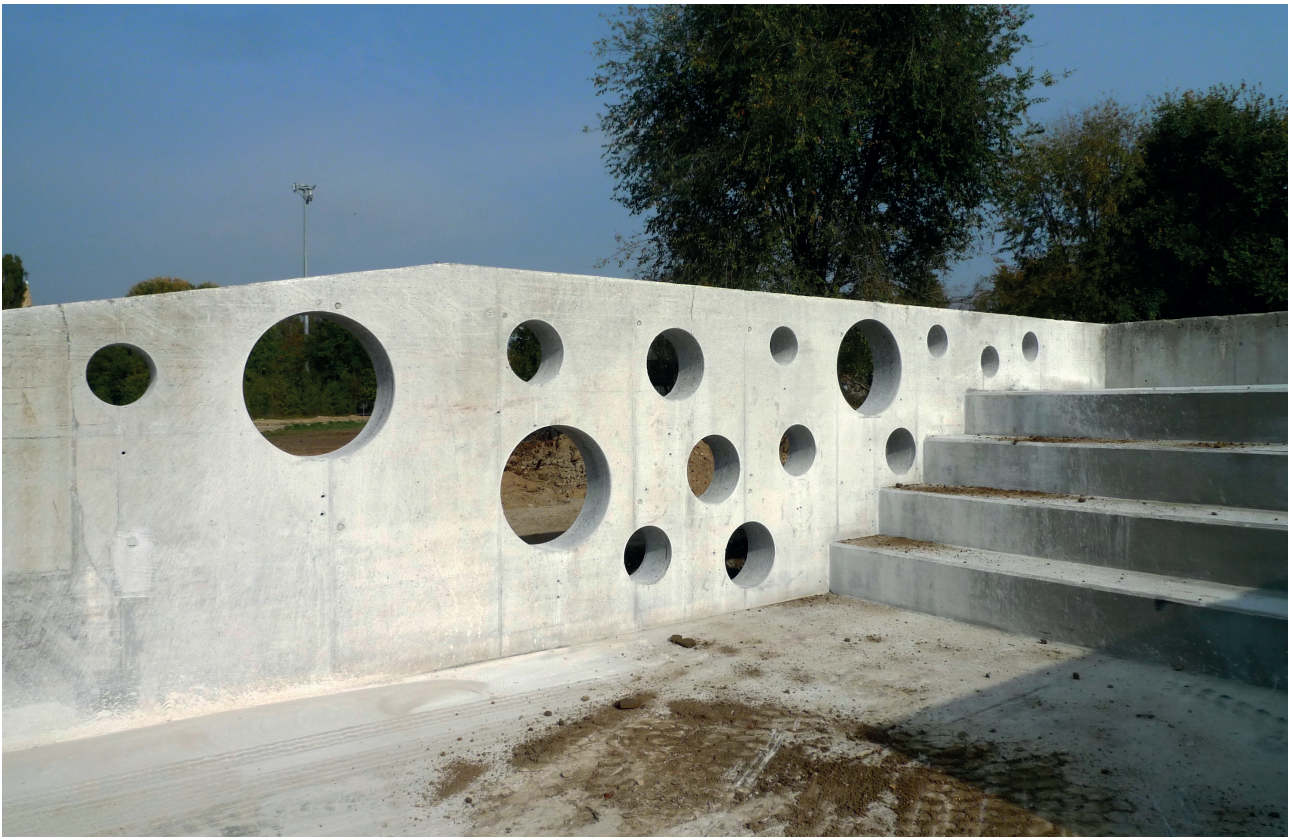
FIGURE 6: Diversified core drilling on the vertical wall.
