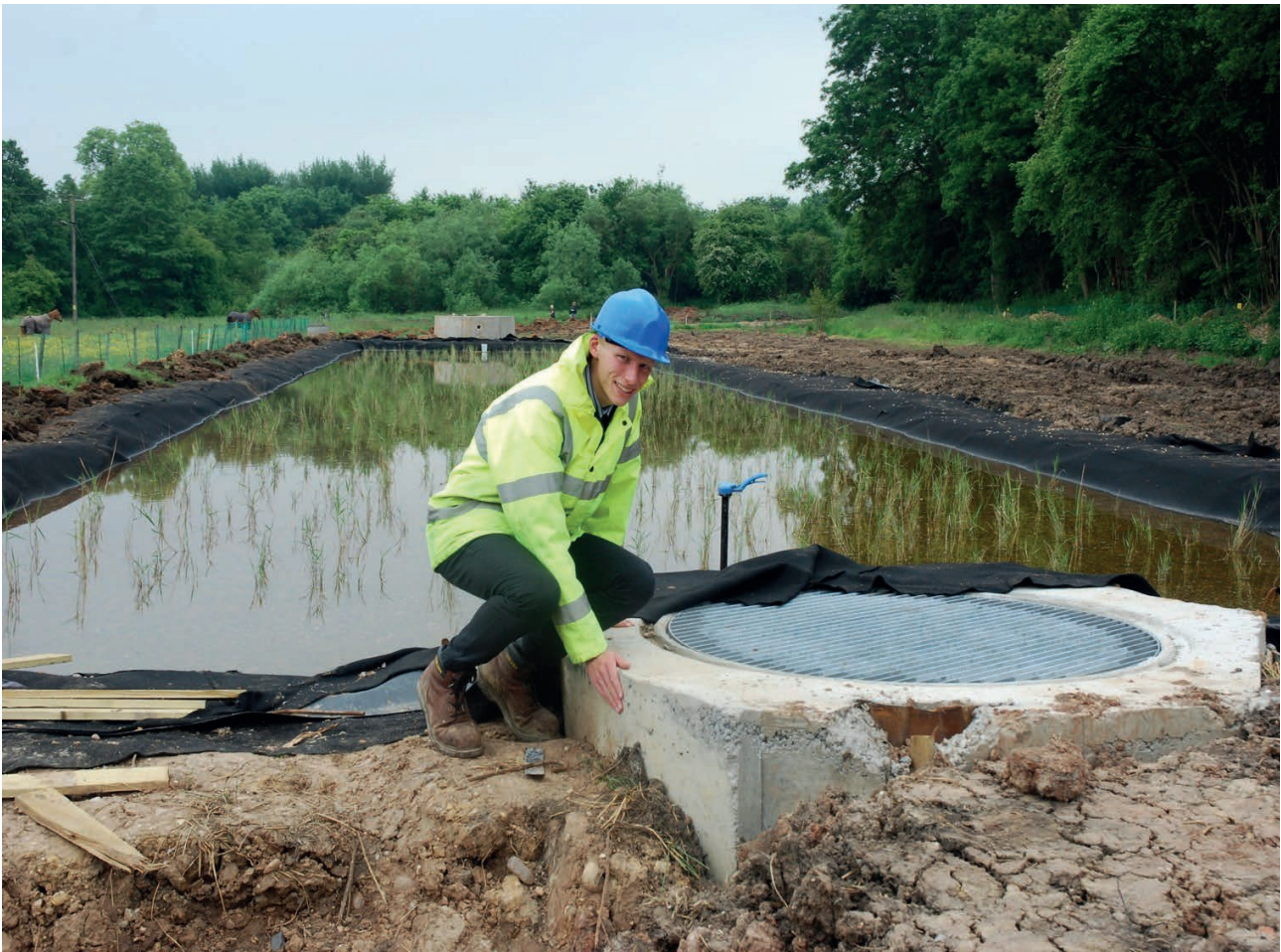
PLATE 1: The chamber at the outlet end of the Shirley Reed Bed during the construction phase of the reed bed
