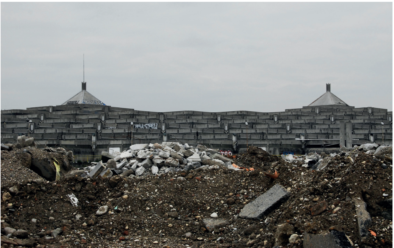
FIGURE 3: The Former Cattle Market ("The Cathedral") of Padua (1965-68), by architect Davanzo, now infrastructure and road waste municipal storage (photo by Stefanos Antoniadis, 2012).
