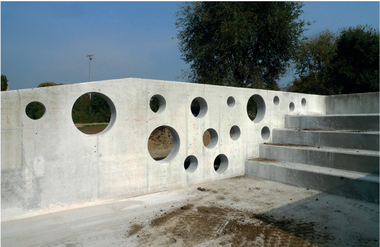
FIGURE 6: Diversified core drilling on the vertical wall.
