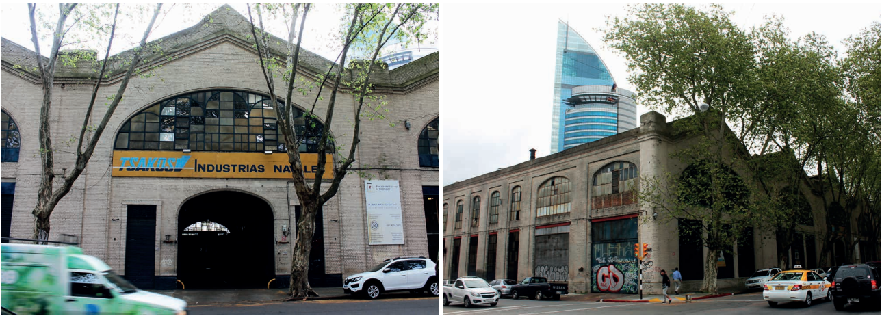
FIGURE 2: View of the Tsakos factory.
