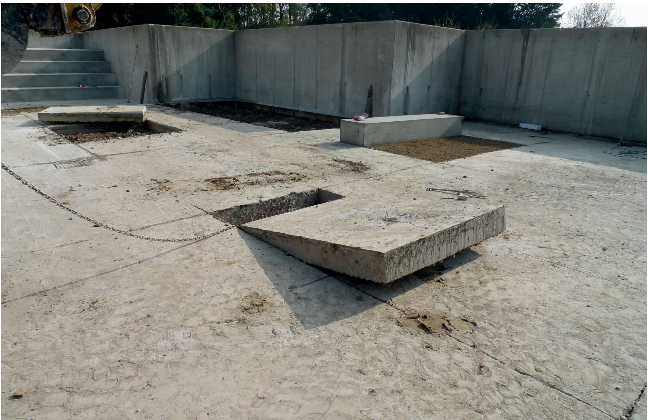
FIGURE 7: Incisions to the ground during recovery of permeable areas.
