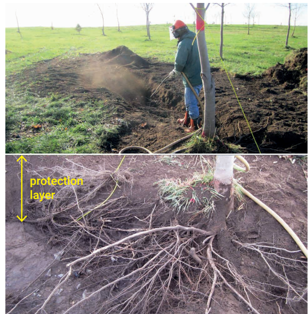
FIGURE 3: Root cleaning with a high-pressure air blow gun (up) and cleaned roots (down) in the protection layer.
