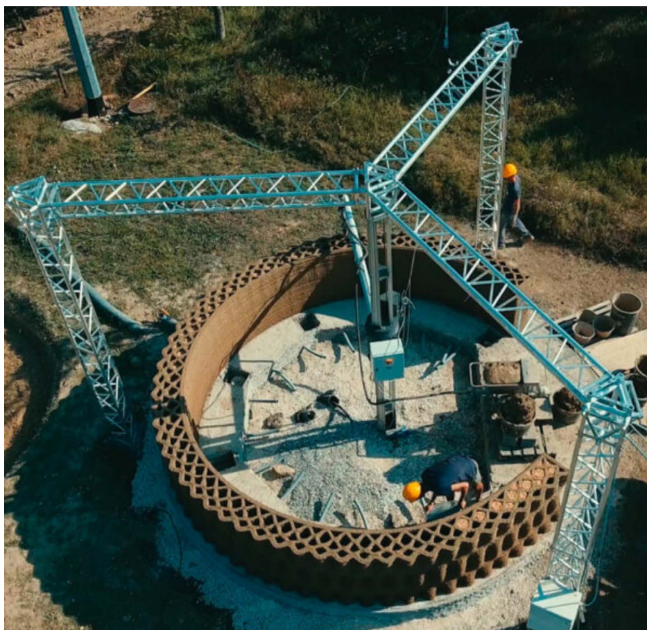
FIGURE 9: Gaia Project by Ricehouse, 3D printed house with biomass insulation built with a 3D Crane WASP printer and natural materials from the landscape nearby, in a blend of natural materials including clay, ground sand, rice straw and rice husk (Source: https://www.ricehouse.it/storie/gaia/ ).
