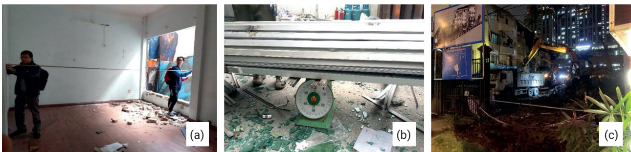
FIGURE 1: Survey of CDW generation (a) Determining GFA; (b) Scrap buyers measuring the amount of aluminum; and (c) Counting the number of CC-CB transport trucks.
