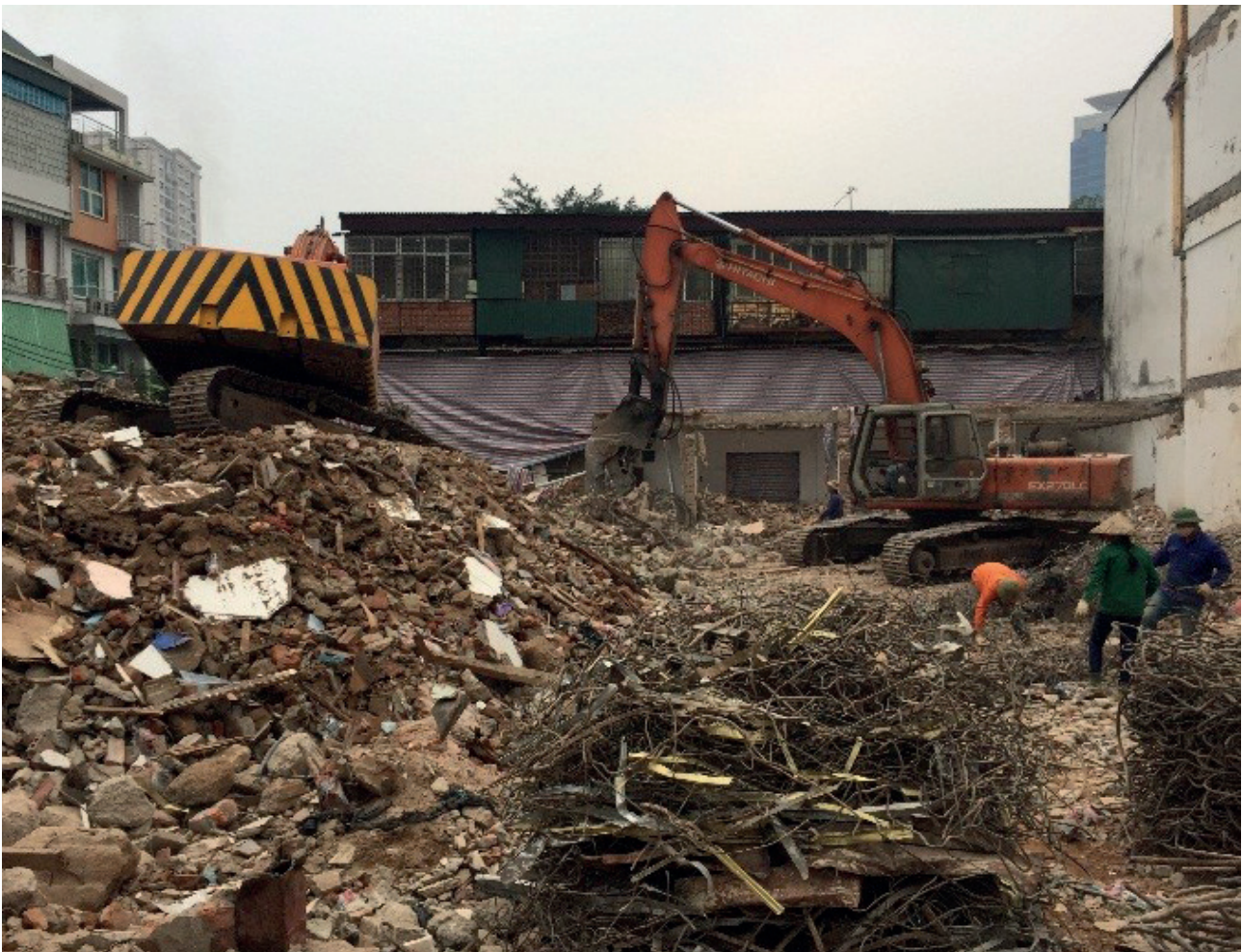
FIGURE 11: Reinforcing steel being separated and recollected.
