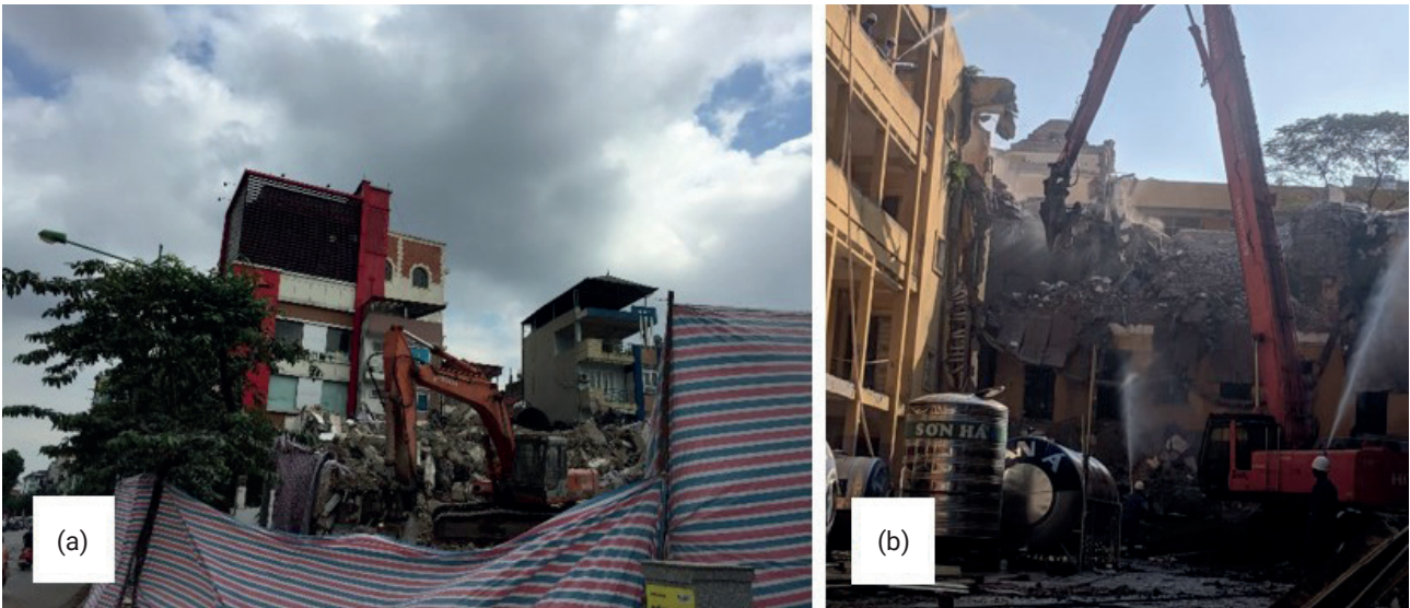
FIGURE 10: Machine demolition at (a) OFC-01; and (b) SCH-01.
