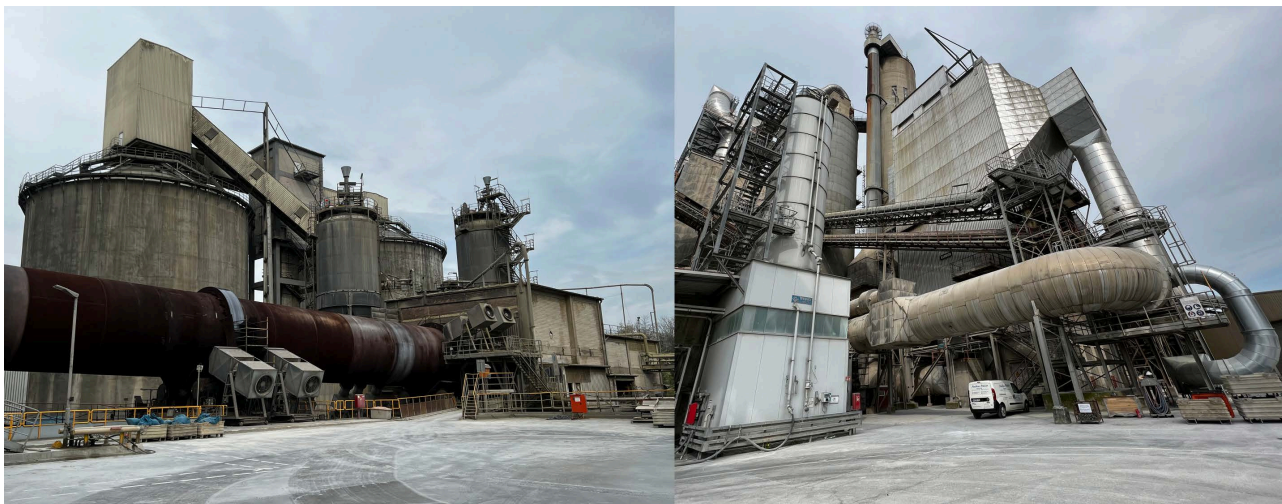
FIGURE 10: Holcim Cement Plant in Beckum, Germany. Source: Author's personal collection, 2023.
