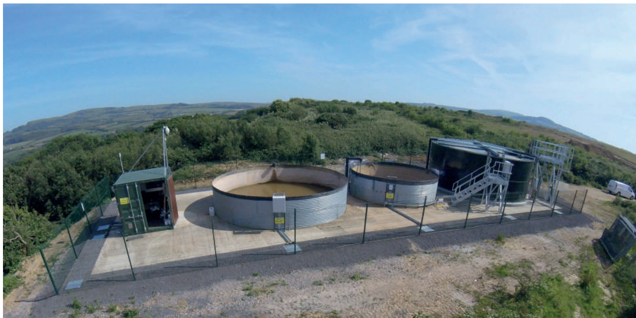
PLATE 1: Aerial photograph of the Bleakdown landfill leachate treatment plant (LTP), showing the control building, RLBT, TLBT, and new glass/epoxy fused steel SBR tank (left to right).
