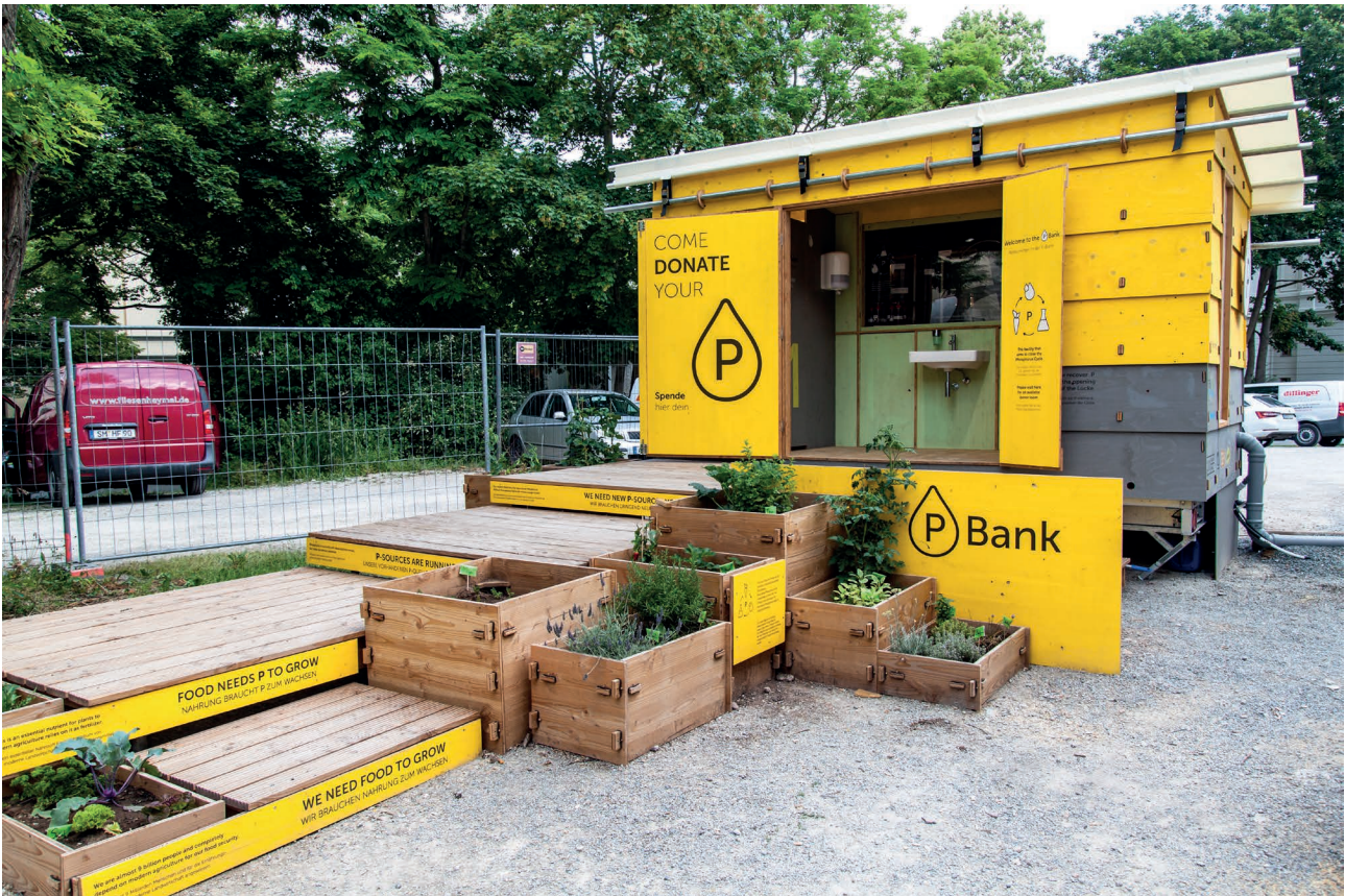
FIGURE 2: Exterior view of the P-BANK on the premises of the Bauhaus-Universität Weimar in 2019.
