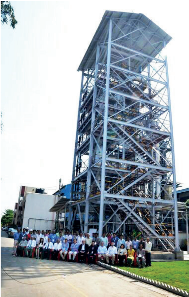
FIGURE 1: 1 MWth circulating fluidized bed solid fuel gasification facility developed during the FP7 OPTIMASH project (2011-2016).
