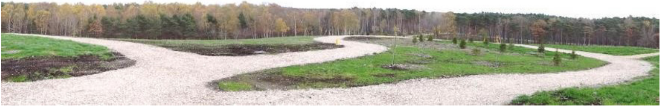
FIGURE 4: View of remediated landfill in 2013 (Tammjärv et al, 2016).
