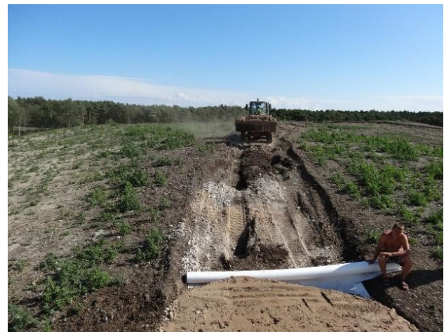
FIGURE 2: Securing trails into soft biocover by supportive geotextile.
