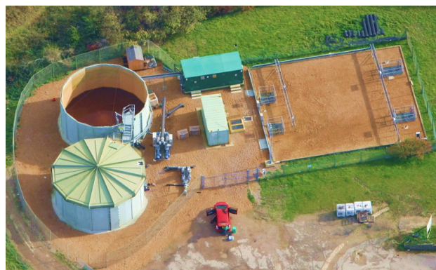
PLATE 3: Aerial view of the updated Small Dole Leachate Treatment Plant, following modifications made in 2010. (Robinson, 2017b).
