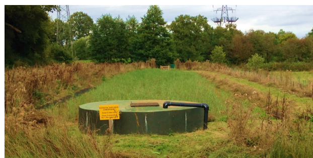
PLATE 1: General view of Shirley Reedbed from the inlet end, showing the Leachate Header Tank in the foreground, September 2014. (Robinson, 2017a).
