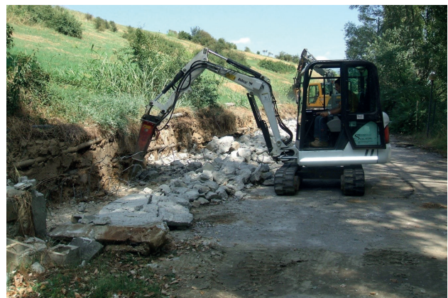
FIGURE 5: Demolition of the perimetric concrete wall.
