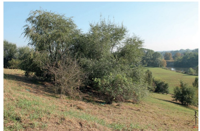
FIGURE 7: The side of the landfill sloping towards the Lambro river.
