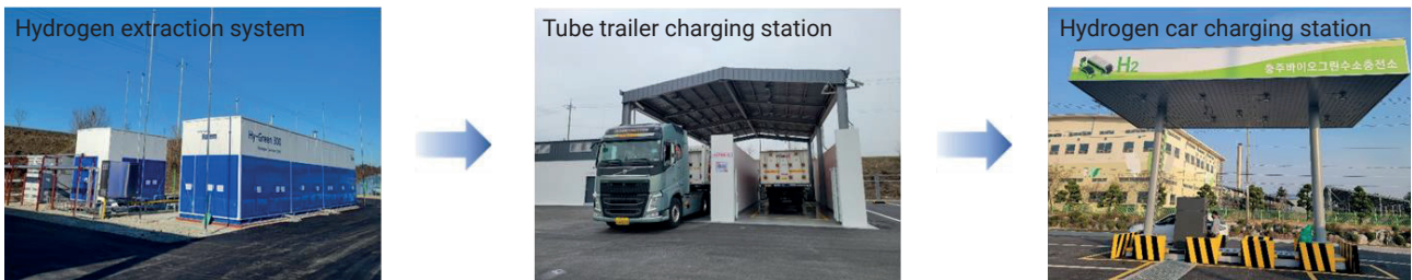
FIGURE 6: The panorama of Chungju Bio Green Hydrogen Charging Station.
