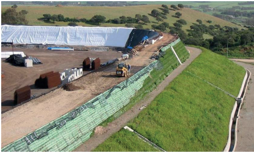
FIGURE 10: Installation of waterproofing liner in the internal side.
