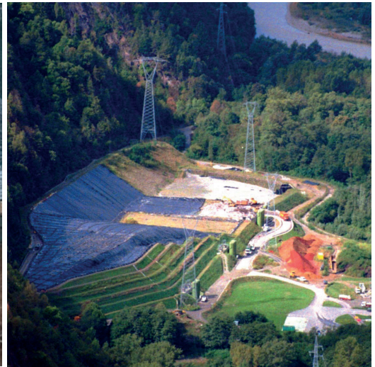
FIGURE 6: Teglio landfill; aerial view.
