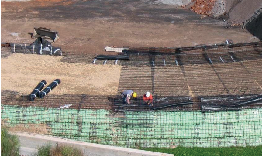
FIGURE 9: Installation of geogrids in Genna Luas landfill.
