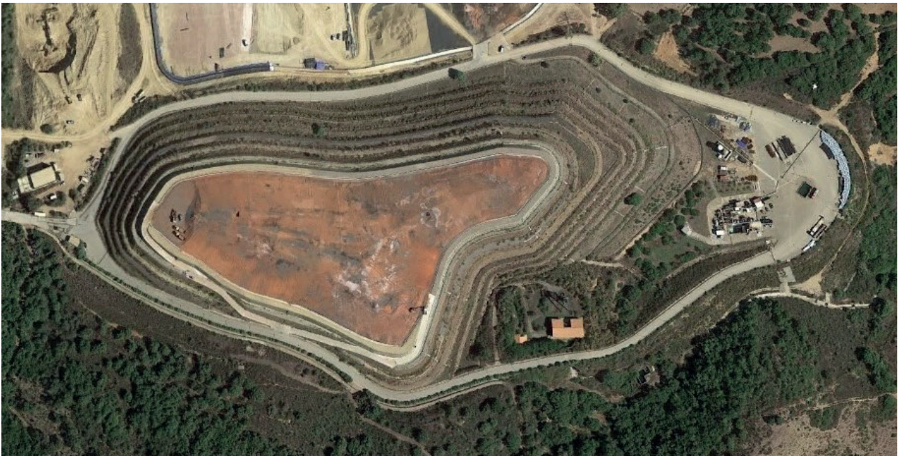
FIGURE 12: Aerial view during construction of the top embankment.
