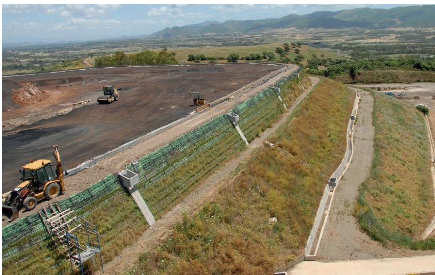
FIGURE 11: Filling phase with ashes.
