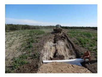
FIGURE 2: Securing trails into soft biocover by supportive geotextile.
