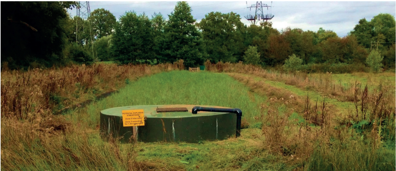
PLATE 2: General view of Shirley Reedbed from the inlet end, showing the Leachate Header Tank in the foreground, September 2014.
