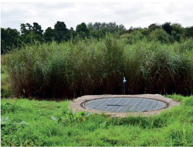
PLATE 4: Outlet end of the reed bed at Shirley during Summer 2016, showing excellent reed growth.
