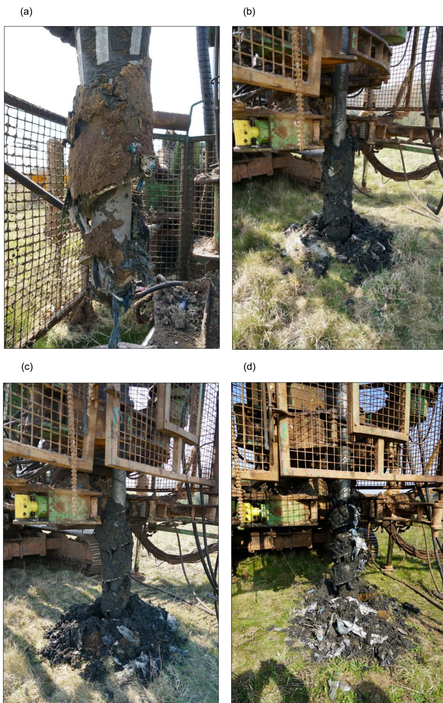
FIGURE 2: Photographs of the recovered wastes from drilling (a) well 1901 (b) well 1904 (c) well 1906 (d) well 1907.
