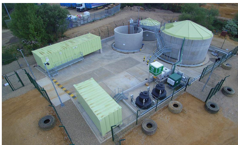
PLATE 1: View of Hatfield Leachate Treatment Plant, showing fully bunded area, chemical dosing compound in right foreground, and control building at the rear left.
