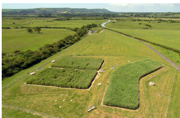
PLATE 2: Aerial view of the vertical flow reed bed, and the two parallel horizontal flow reed beds, following construction by Phoenix Engineering in 2010.
