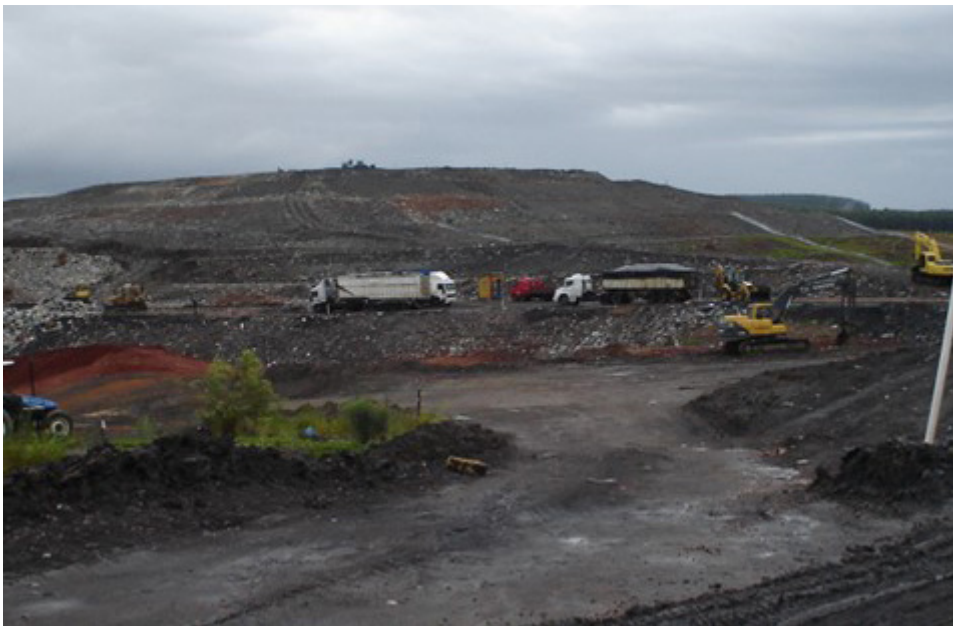
FIGURE 2: A daily service front of the landfill.
