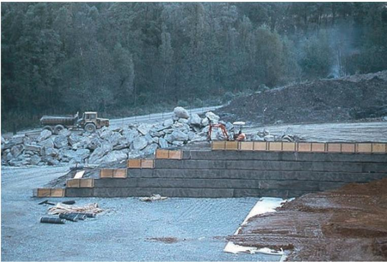
FIGURE 5: Teglio landfill; internal side of the landfill (compacted clay layer can be seen).
