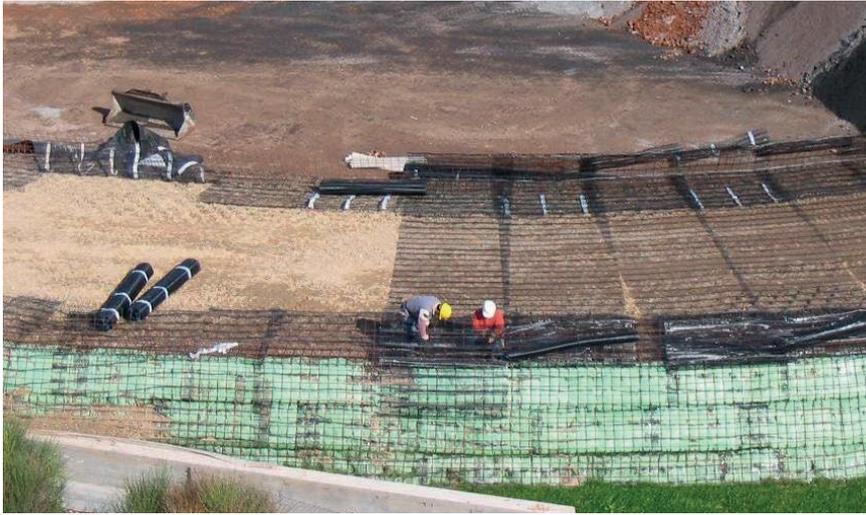
**FIGURE 9:** Installation of geogrids in Genna Luas landfill.
