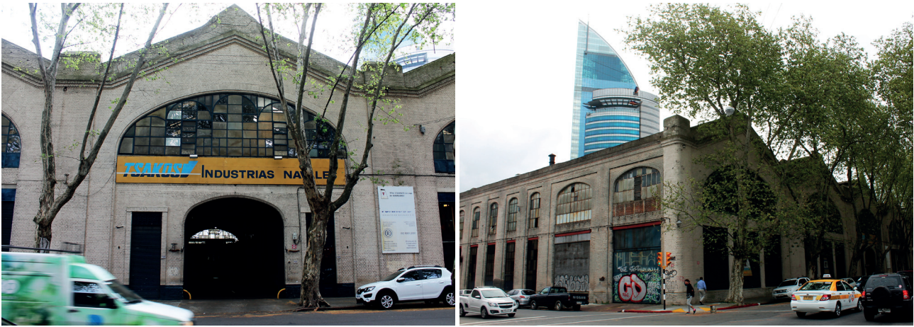
FIGURE 2: View of the Tsakos factory.
