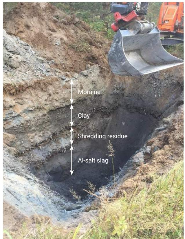
FIGURE 4: Landfill layers at the Vierumäki industrial landfill.
